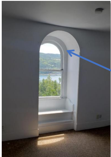
EXISTING LEVEL 3 DORMER BEFORE RENO
