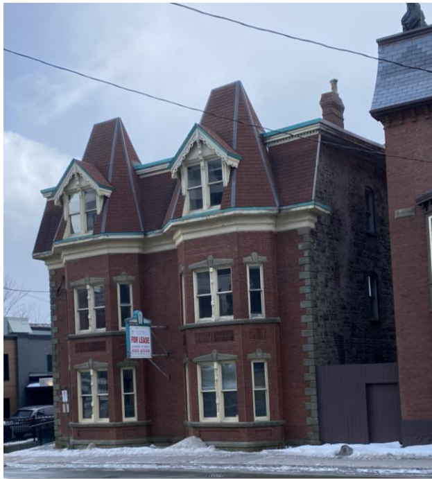
EXISTING FRONT OF DEVON HOUSE WITH BAY WINDOWS EXTENDING INTO THE MANSARD AND TRADITIONAL BAY WINDOWS ON DEVON ROW.
