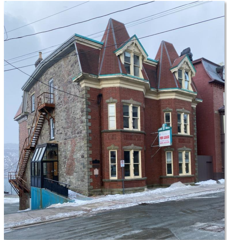
PUBLIC VIEW OF DEVON HOUSE FROM DUCKWORTH STREET
