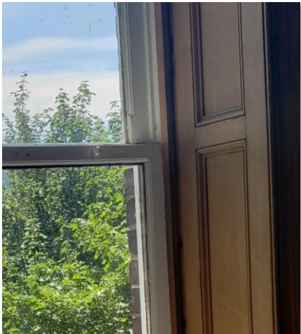
EXISTING STAIRCASE WINDOW AND INTERIOR TRADITIONAL PANEL DETAILING
