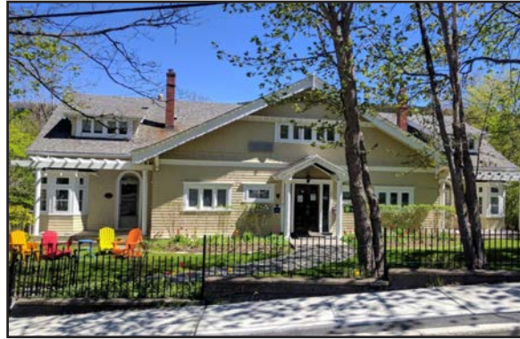
Prominent Front Facing Gable Steeply Pitched Gable Roofs
