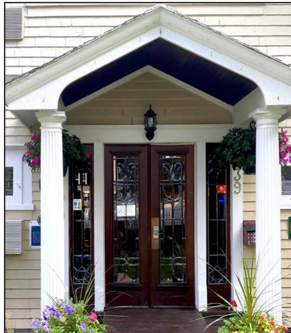
Deep, open porch supported by wooden columns, main wooden door with leaded glass insert and light
