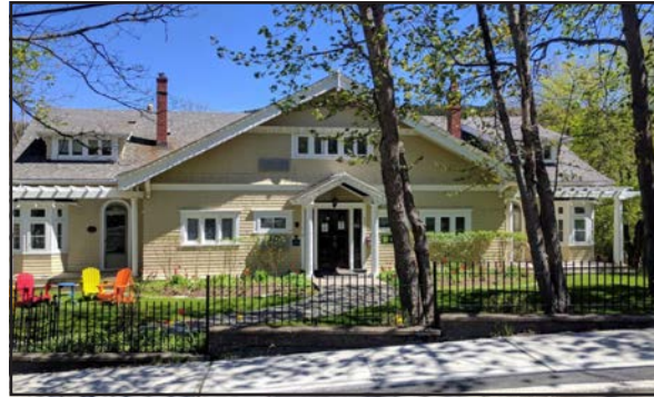
North facing/ Main facade
