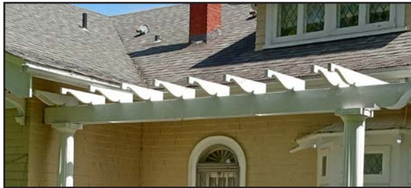
Projecting wooden eaves
