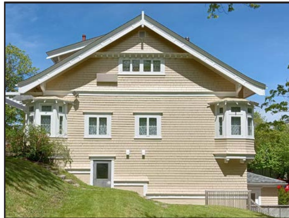
West facing facade
