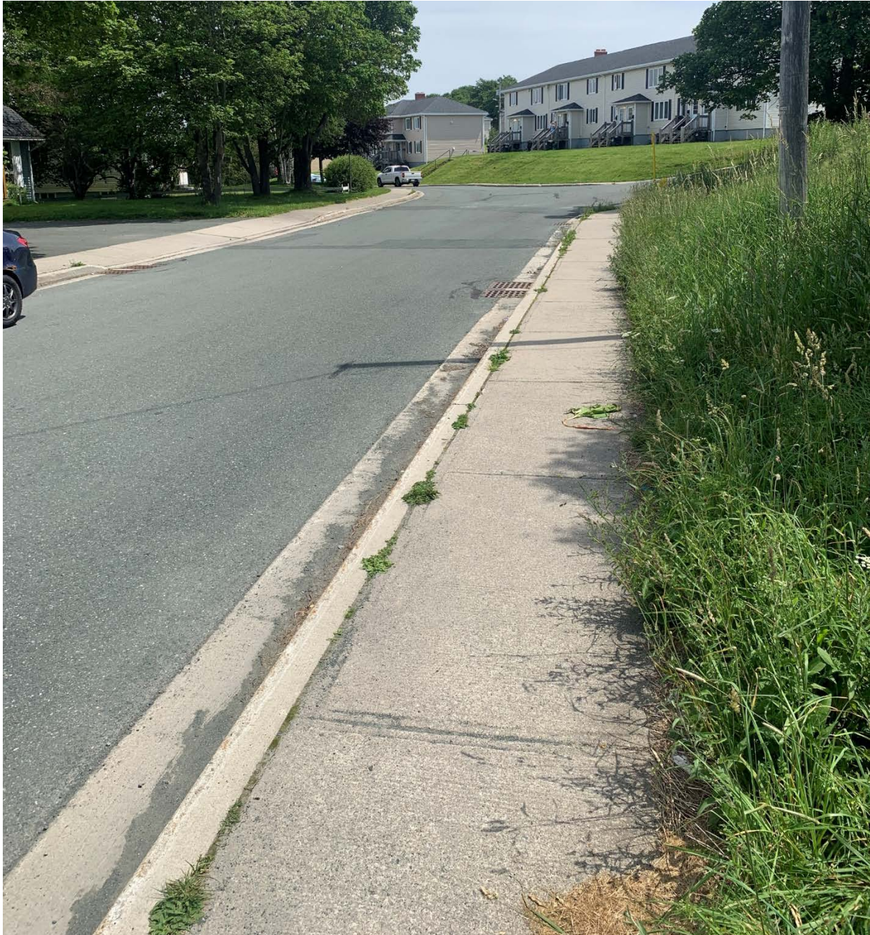
Figure 5: Site Access, Sight Line East of Access (Looking to the Right)
