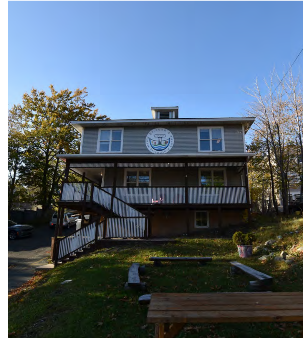
Street-Facing Facade of 716 Water Street showing lacking parking, inaccessible entry
