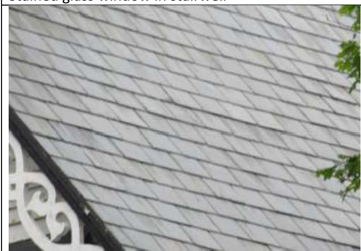
Bargeboard and slate roof
