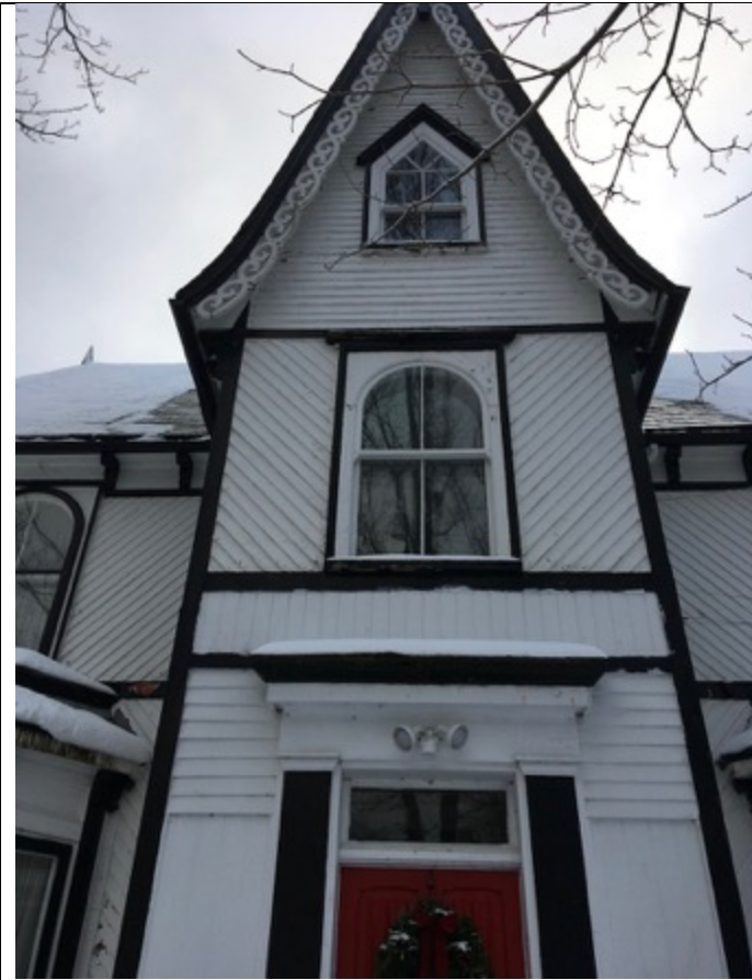
Siding, bargeboard, and window details (East side)
