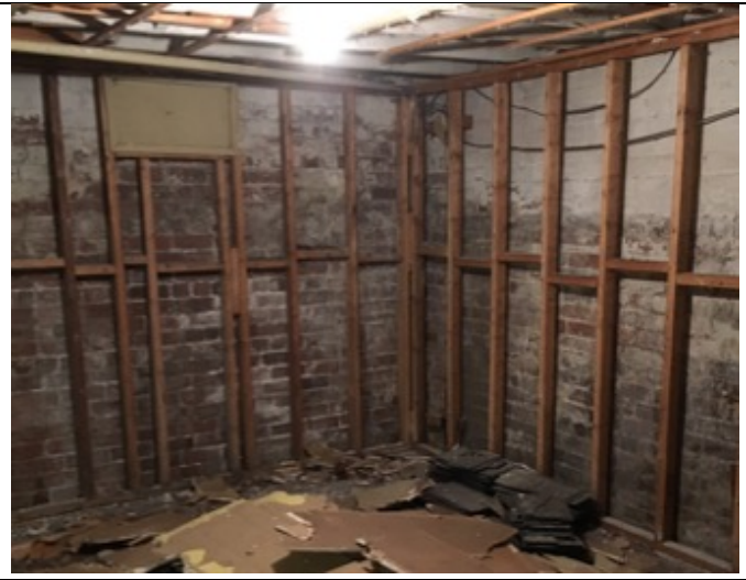
Brick foundation walls in Northeast corner
