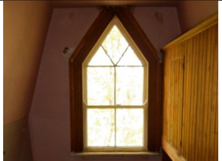
3 rd floor, double-hung gothic window (middle, East)
