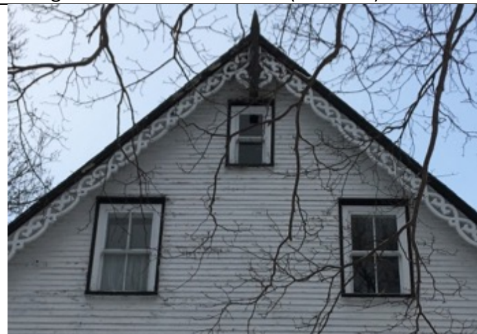
Bargeboard and window details (South side)
