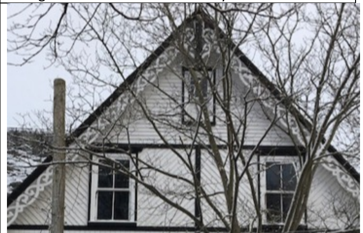
Bargeboard, windows, and siding details (North side)
