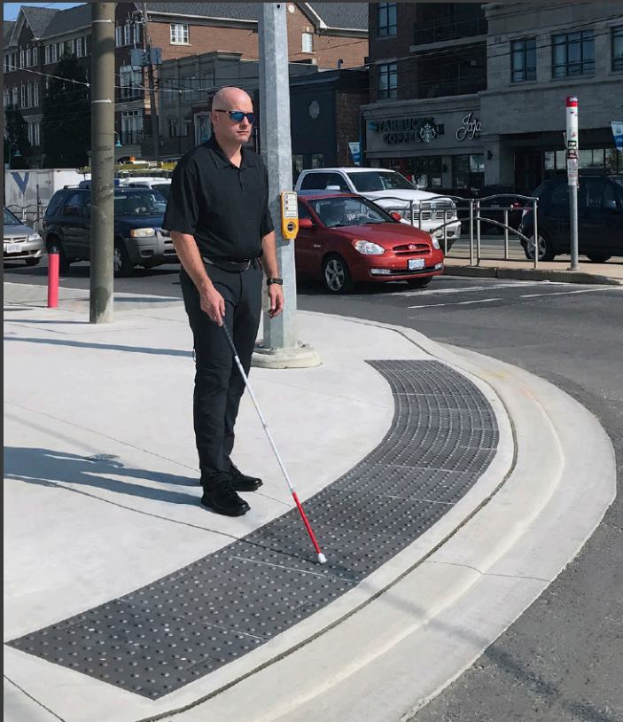
Tactile wayfinding surface indicators are textured surfaces embedded in sidewalks which inform visually-impaired users that they are approaching an intersection or crosswalk. These should be provided at all crossing locations in Churchill Square.
