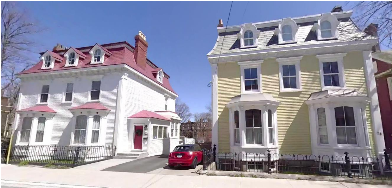
Buildings located at 30 and 28 Monkstown Road.
