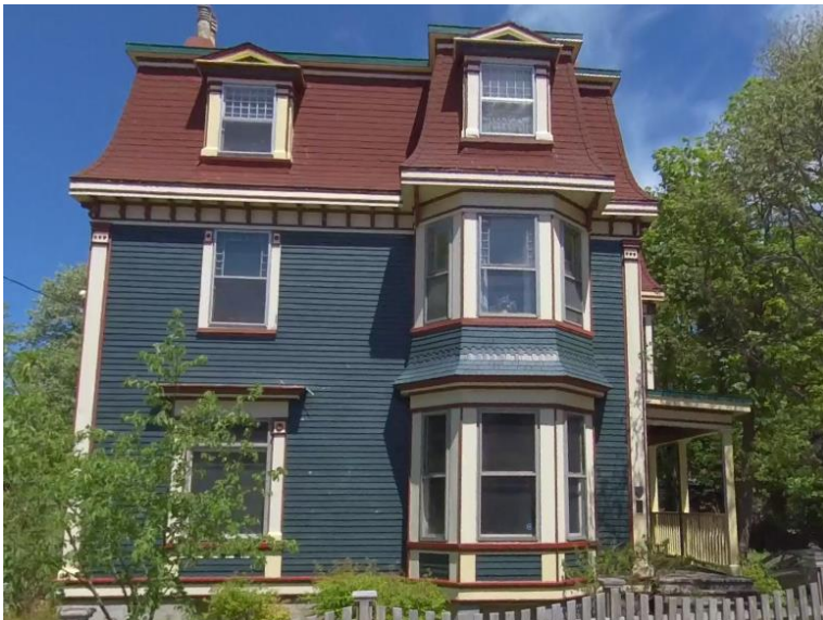
Heritage Building located at 36 Monkstown Road.
