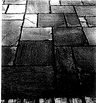
Plate 13: Chisel cut natural flagstone patio example.
