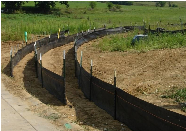
Figure 10-12 - Silt Fence
