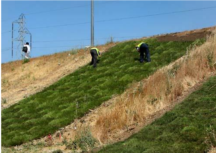
Figure 10-2 - Temporary Grass and Permanent Vegetative Cover
