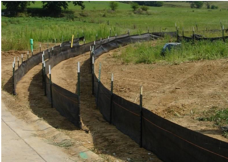
Figure 10-12 - Silt Fence
