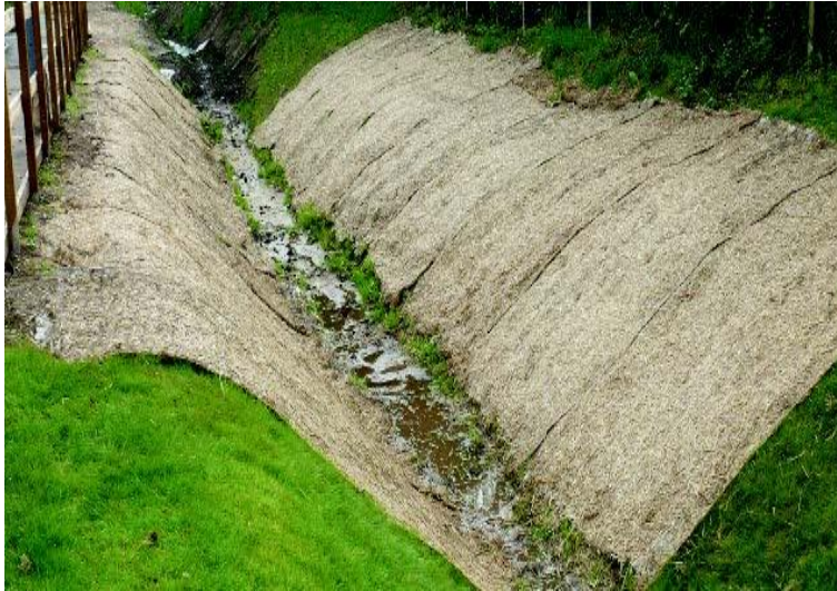
Figure 10-4 - Erosion Control Blanket
