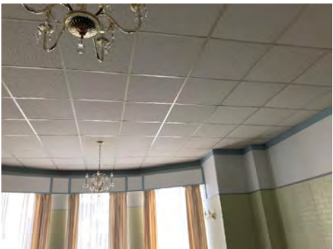
Typical drop ceiling over drywall or plaster
