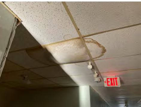
Fairly isolated occurrence of water damage
